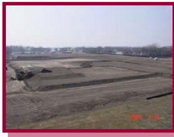
Site pictures from Friday March 18, 2005 showing the removal of the surcharge soil from the building pad.
