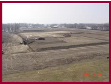
Site pictures from Friday March 18, 2005 showing the removal of the surcharge soil from the building pad.
