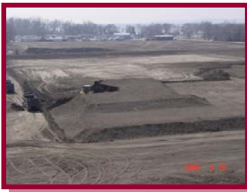
Site pictures from Friday March 18, 2005 showing the removal of the surcharge soil from the building pad.
