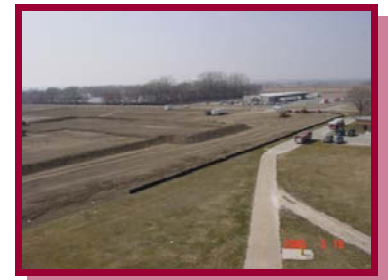
Site pictures from Friday March 18, 2005 showing the removal of the surcharge soil from the building pad.
